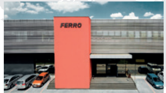
FERRO headquarters in Skawina
